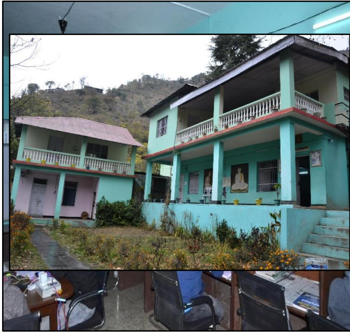
1 st building left side and library and rooms
